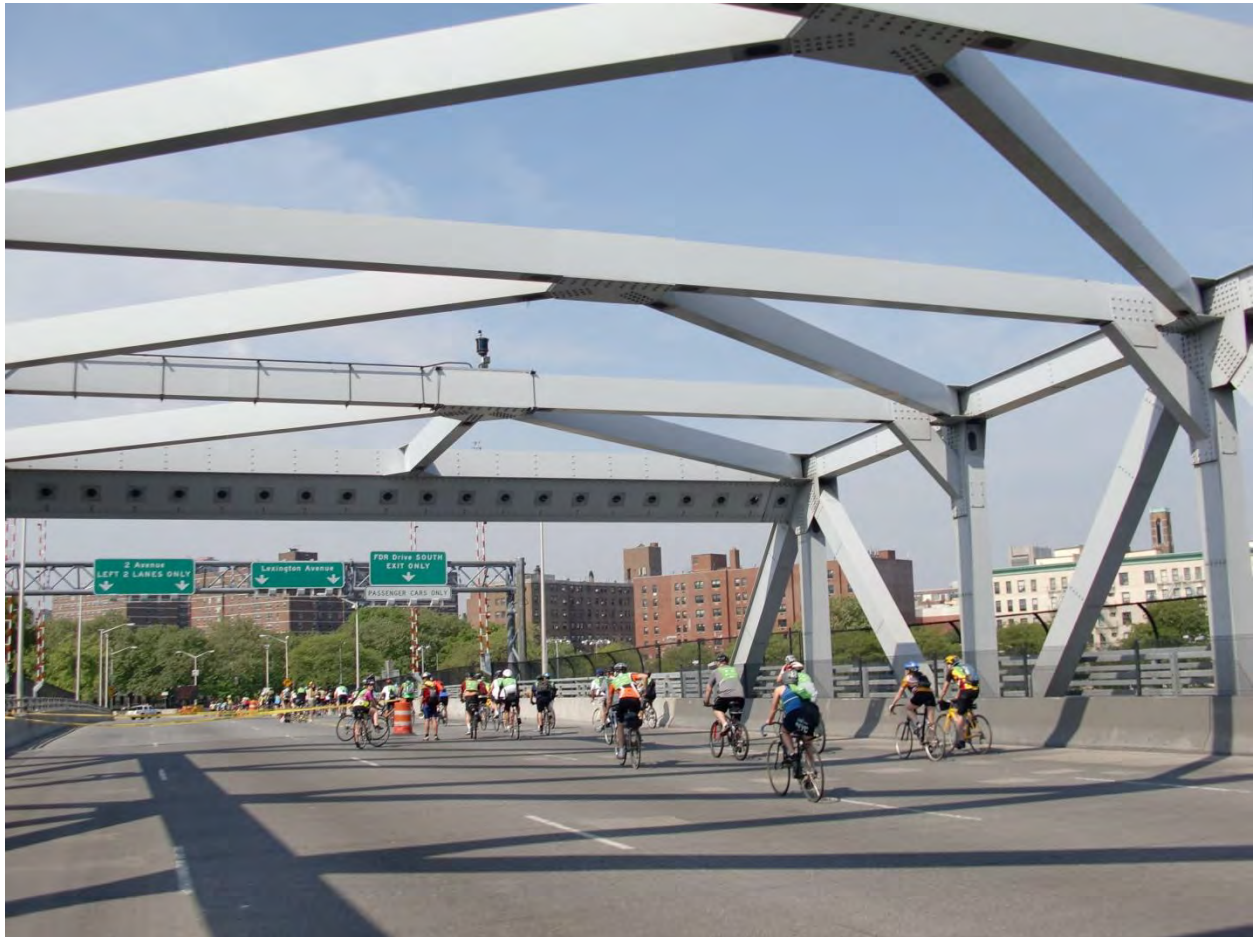
Crossing one of the bridges along the route
