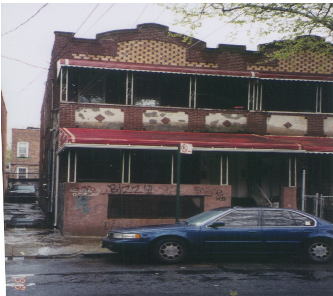
619 Vermont Street, Brooklyn New York (Picture taken about 2002)
