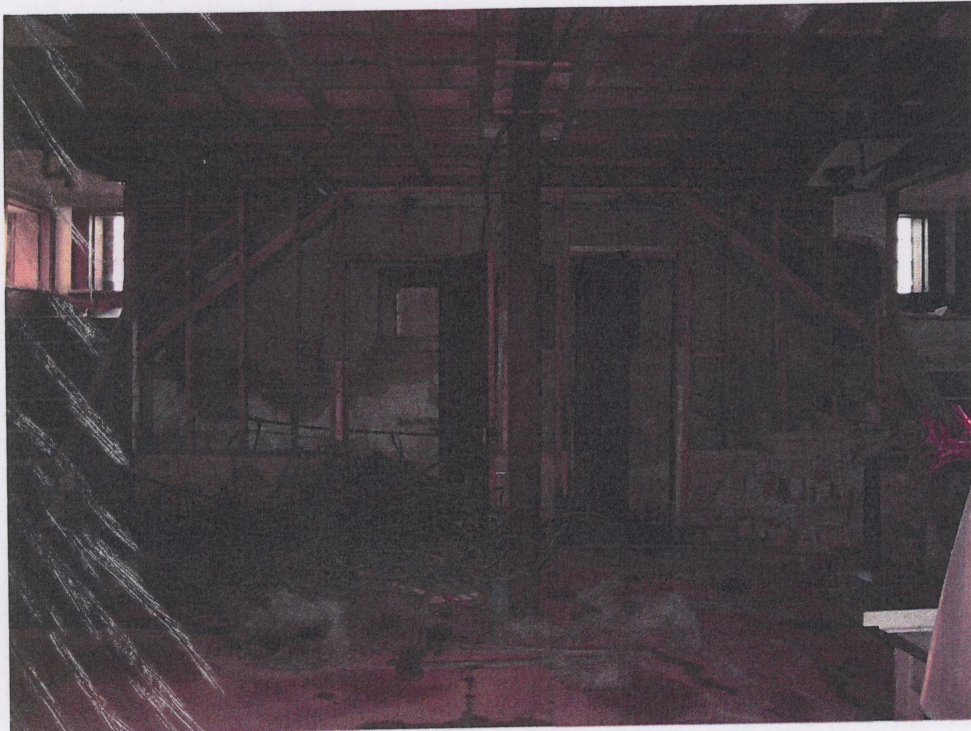
19: View from Basement looking back toward stairs
