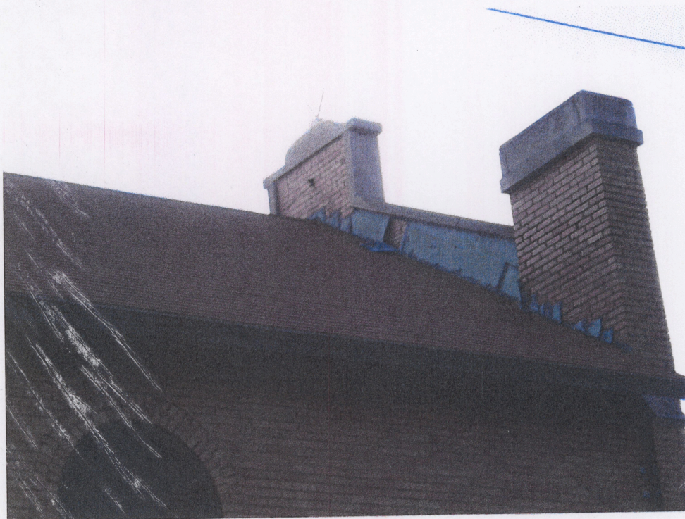
E6: Condition of front parapet from rear
