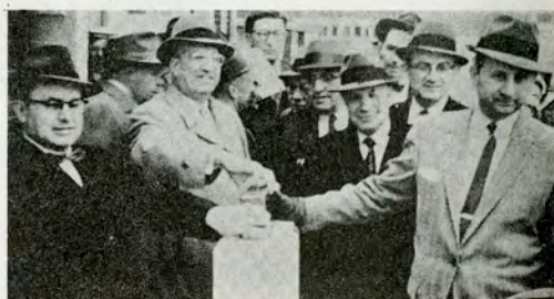
PREPARING THE CORNERSTONE
