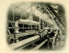
This central station power plant contract provided for the piping for 4 boilers (300-lbs. 160 degrees superheat), 2 turbo-gen-
