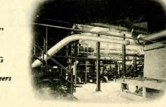
This piping installation included all power house piping for eight boilers (250-lbs. 125 degrees superheat) and three 10,000 k.w. turbo-generators. In addition, all incidental and
